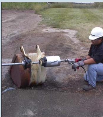
Step 3: Attach the drill and start boring
