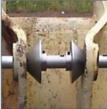
Step 1: Center the boring bar
